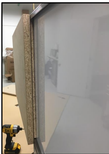
Sliding front onto refrigerator
